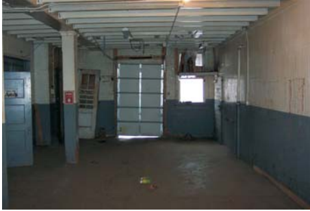
FIRST FLOOR BEFORE
