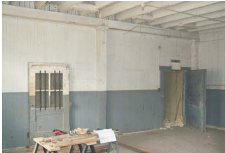
SECOND FLOOR BEFORE
